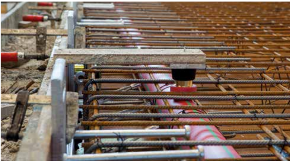
Prefabrication concrete wall
