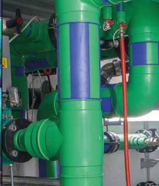
Welded connection PP-R
