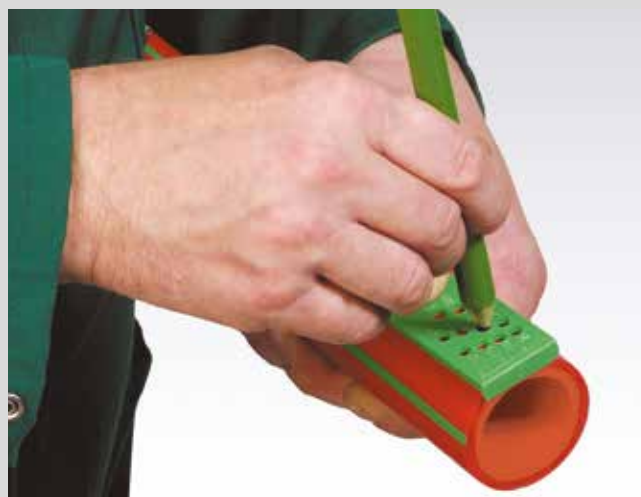
Marking of the welding depth
